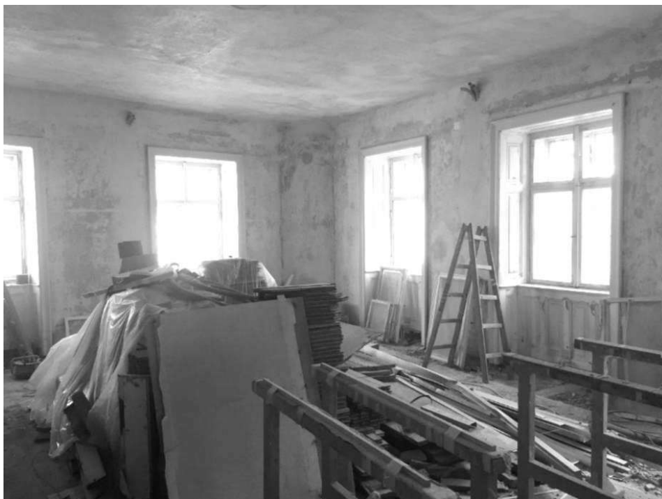
Figure 6: The new office premises under construction (Photo courtesy by L. Thrainer).
