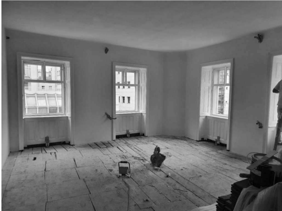
Figure 14: The open-space office under construction, before... (Photo courtesy by L. Thrainer).
